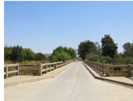
Bridge over the Orange River
