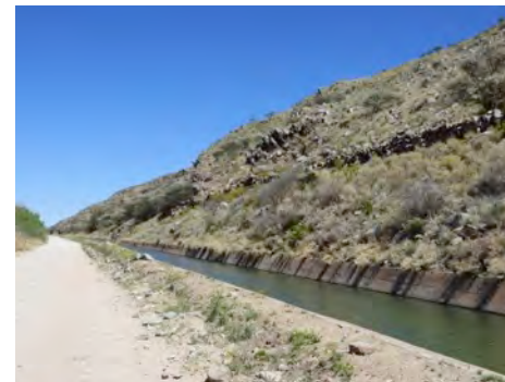
Orange River Canal System
